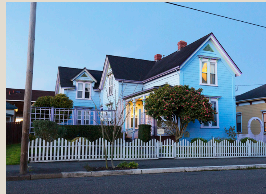
The historic Sarah Carson House (above) is one of three underused buildings in Eureka that will be
